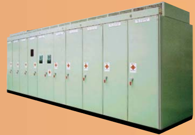
2007 30MVA IGBT Drives for steel rolling mills delivered
